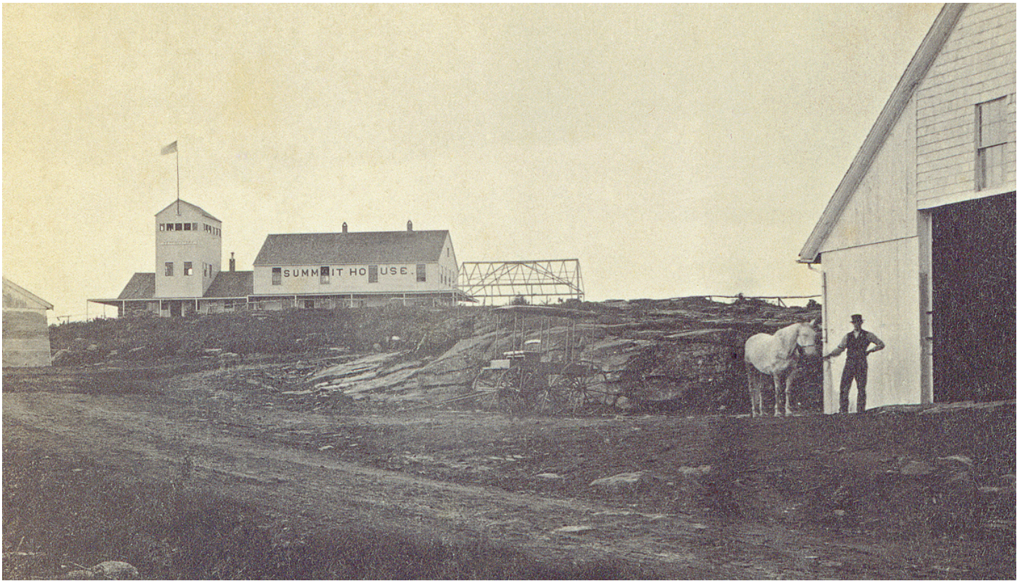
Summit House I - After Expansion With Barn
