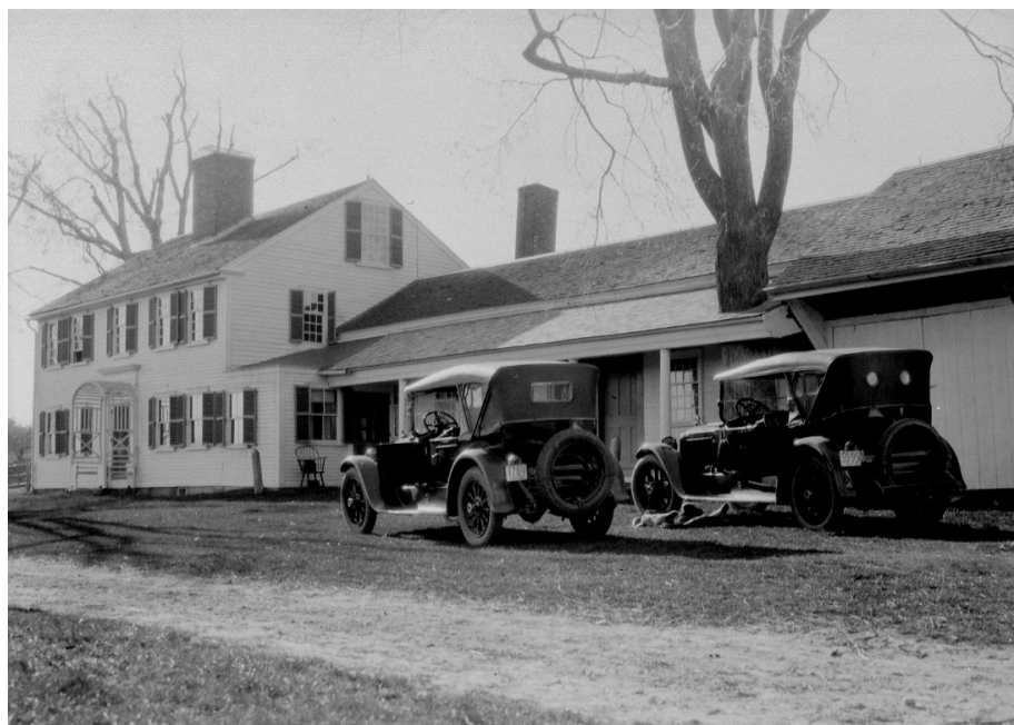
Early 1930s - note tree through porch roof
