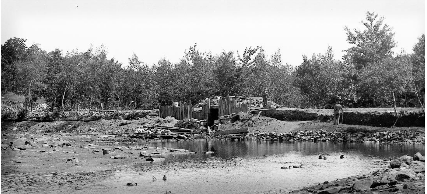
Replacement Dam and Spillway Being Built in 1905
