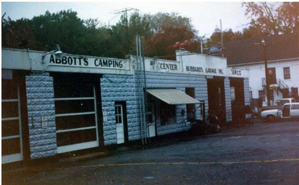
The garage as it looked near the end in October 1979
