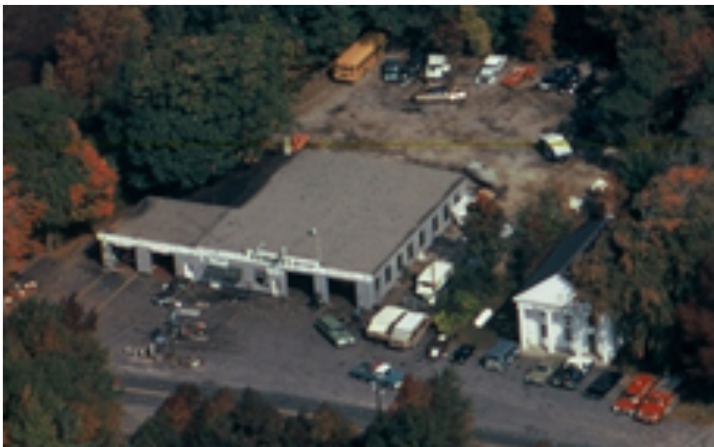
Notice the 2 Bays on the left end, which once housed a fire engine and an ambulance. Today, they have been converted into convenience store.
