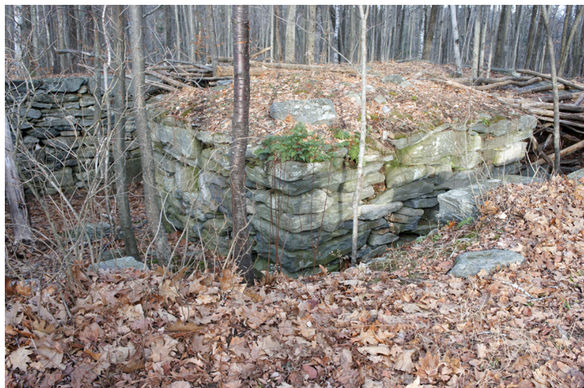
Center Chimney Foundation 12/2021
