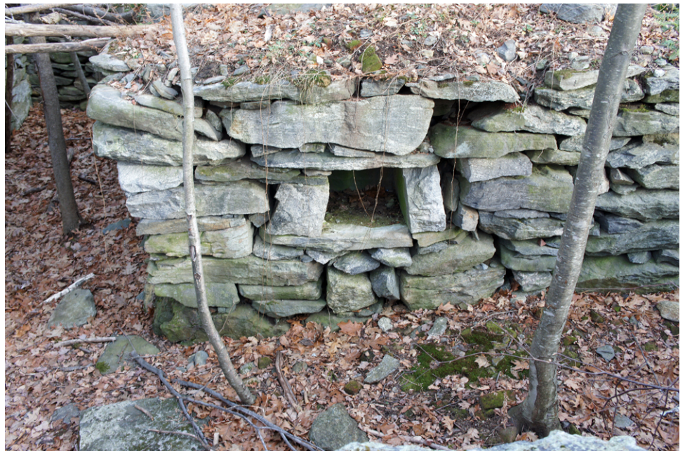
On all 4 sides of the chimney base in the cellar there appears to be a Firebox. Was that to provide heat for boarders who slept there?
