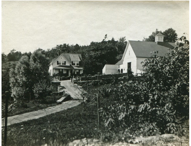
Silas Fay Farm at 19 Allen Hill Rd.
