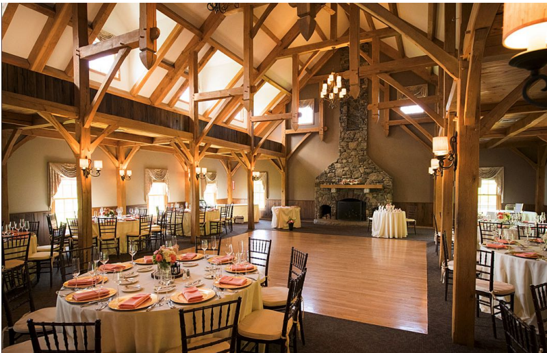
Post and Beam Banquet Hall Addition
