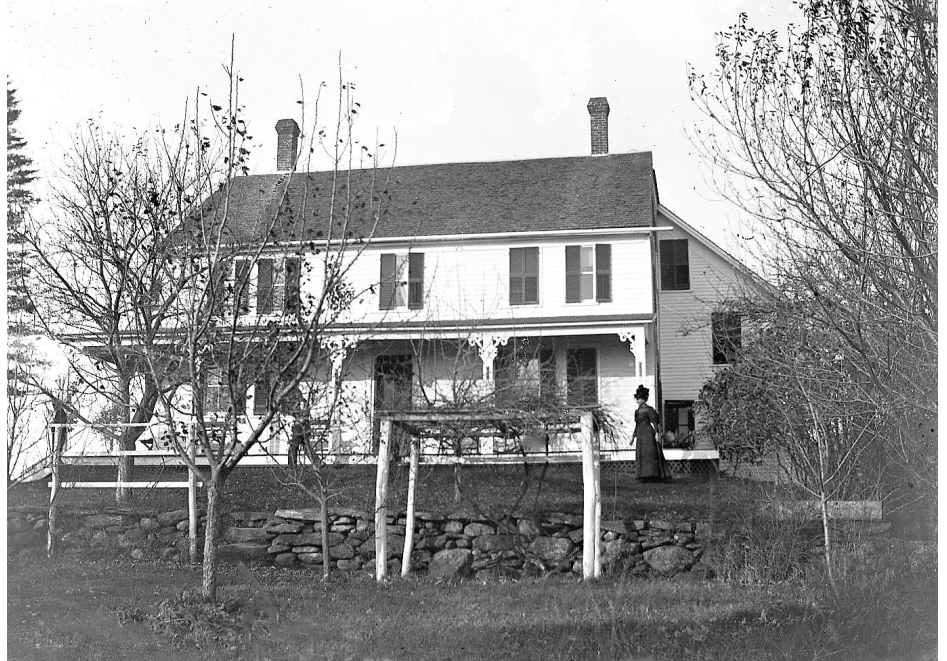
Original Harrington Farm Before Renovations Without Dormer and Read Addition
