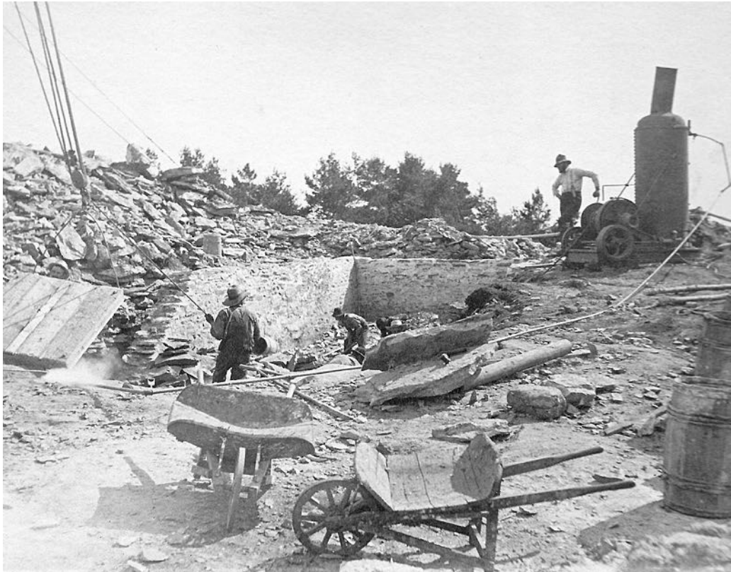
Foundation Construction With Blasted Rocks All Around
