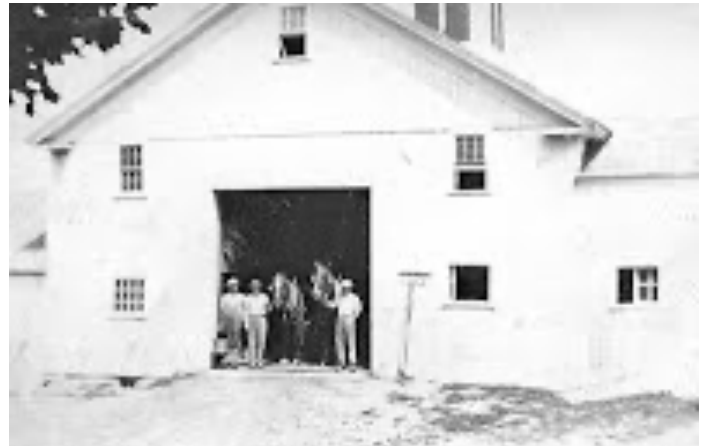
Barn on east side of Worcester Rd. Facing the house
