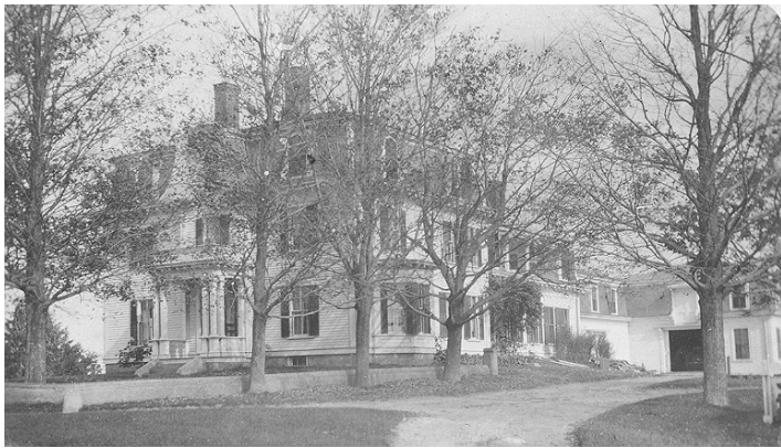
House and Horse/Carriage Barn early 1900's
