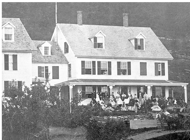
The Right-Hand End of this building was the original farmhouse and it was expanded numerous times.
