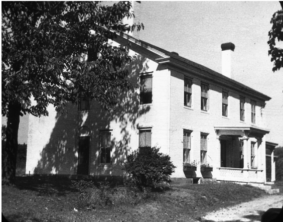
House on west side of Worcester Rd. Facing East
