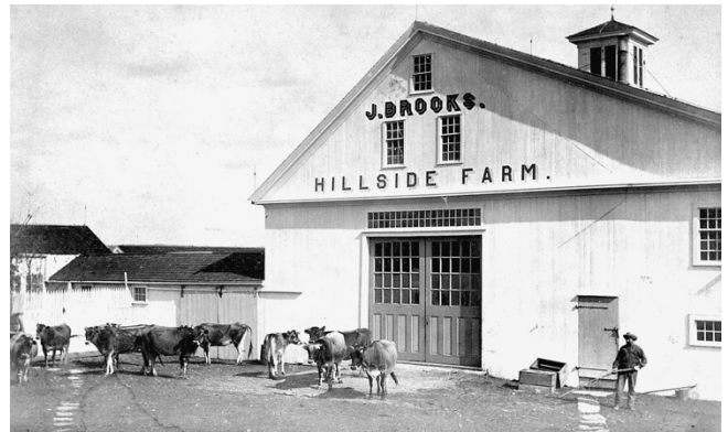
Barn for Hillside Farm, aka. John Brooks Farm
