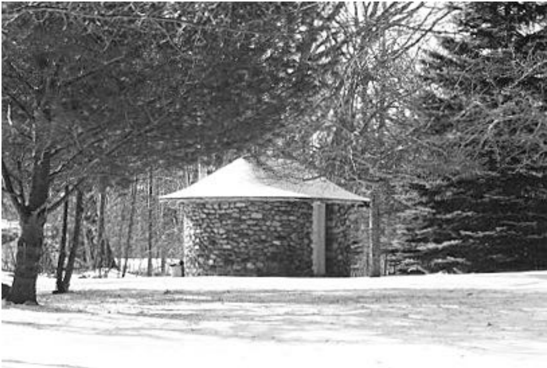
Minns Well House, 38 Radford Rd. (1912) - Photographed by Joyce Anderson
